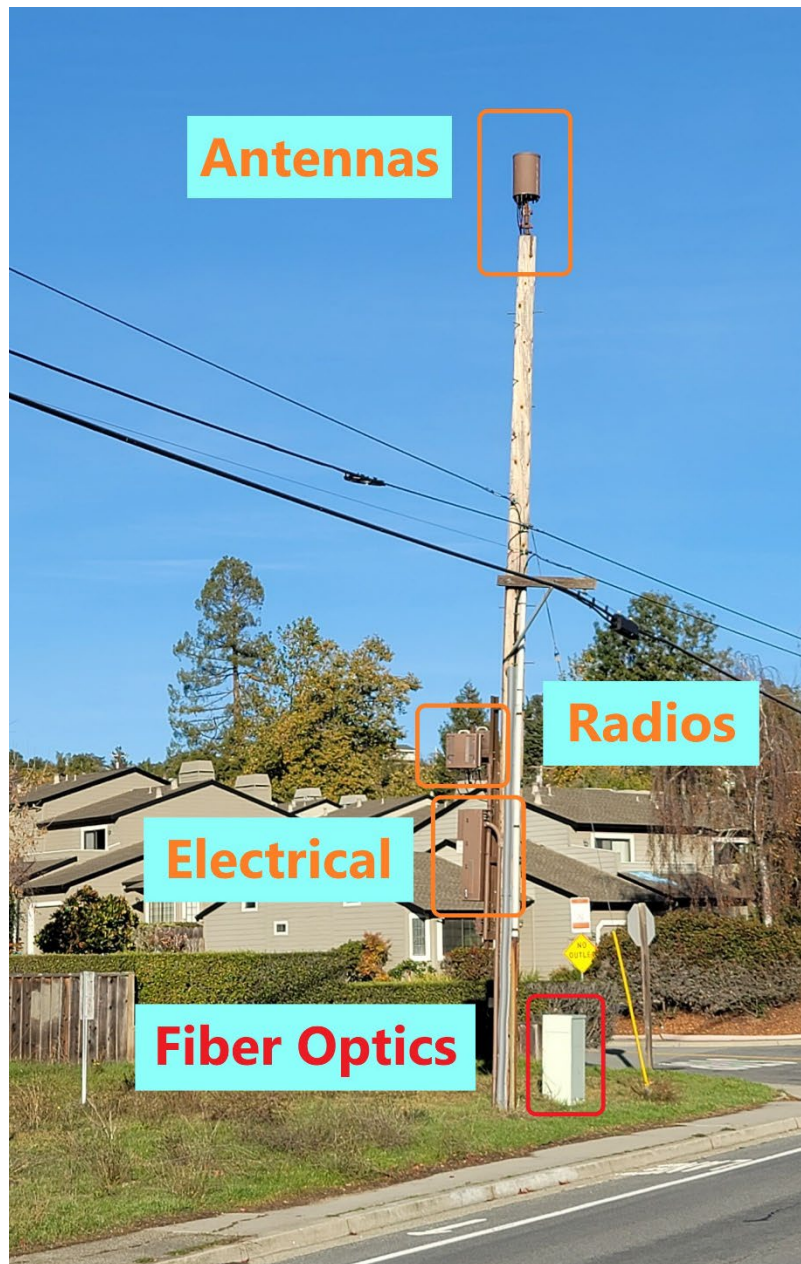
Figure 2. Components of a Small Cellular Site (Photo/Edits by David Witkowski)
